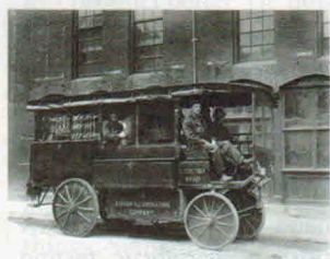
Detroit Edison's electric overhead line truck, 1915
